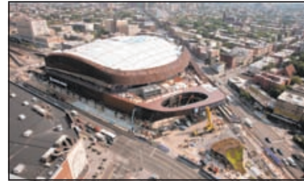
AUG. 23, 2012: What a beaut! With the roof finished, logos gleaming from the sides. The venue is nearly ready.
