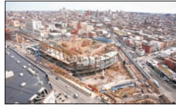
MARCH 25, 2011: Up it goes! The Barclays Center's skeleton-like frame rises into the air on two sides.
