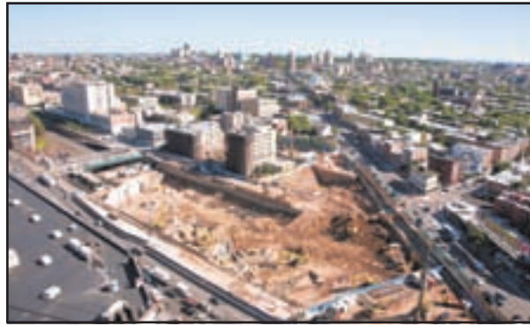
AUG. 30, 2010: A fleet of backhoes make some progress in the construction crew's frantic quest for bedrock.
