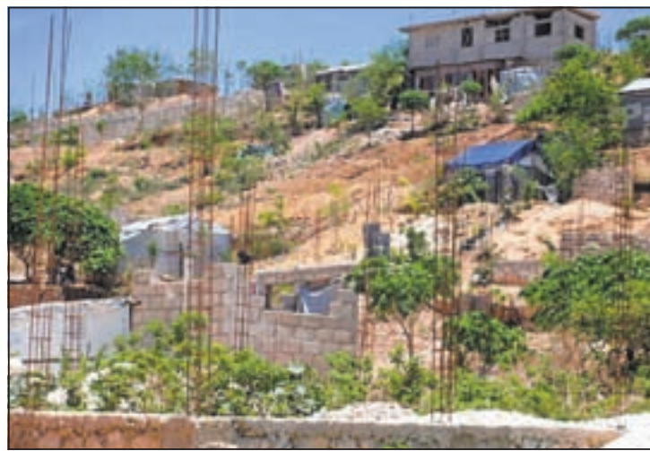
A typical Canaan hillside, with many houses under construction. HGW/Milo Milfort
