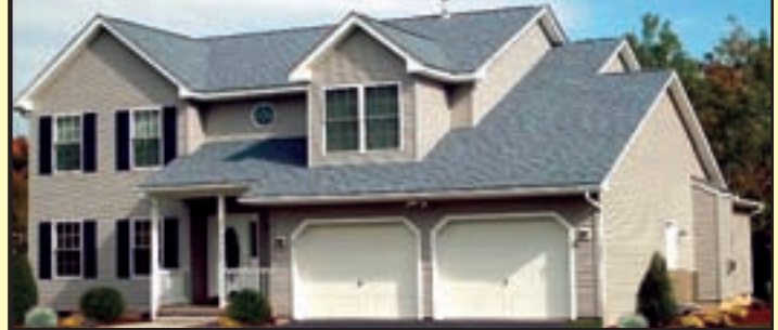
THE ASHTON -- A Classic Mainline Home
