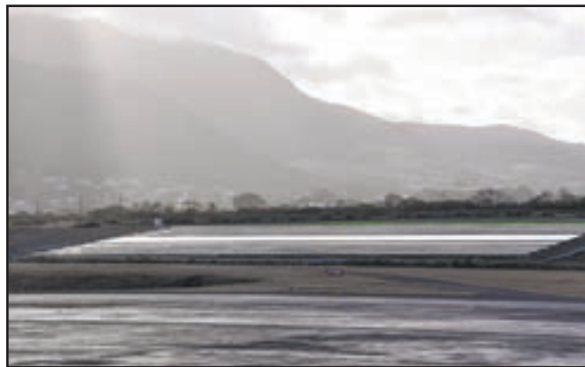
St. Kitts and Nevis has launched a 1-megawatt solar farm at the country's Robert L Bradshaw International Airport. A second solar project is also nearing completion.
