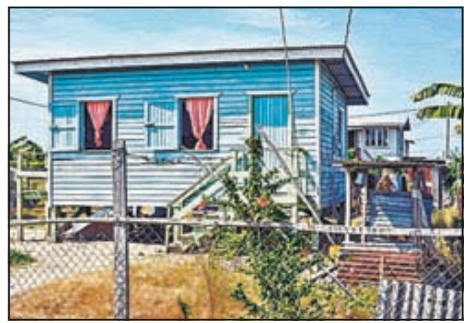
One of the houses built for Mahaica residents who relocated to Hope Estate in Guyana. Inter Press Service / Samuel Maughn
