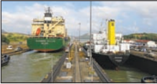
Two ships go through the Miraflores locks on the Pacific side of the Panama Canal, which raise or lower vessels 16.5 metres and take 40 minutes to pass through. Inter Press Service / Iralis Fragiell
